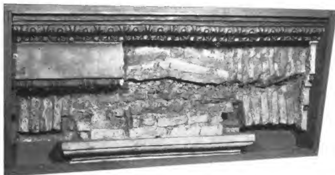
Fig. 40. S. Maria Maggiore, Nave architrave, springing of relieving arches, flat brick arches and eighteenth century patchwork (from plaster cast)
